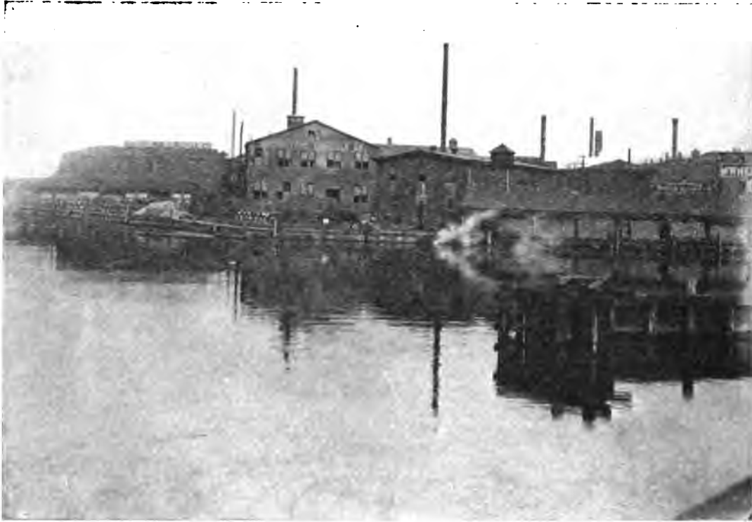
East Shore Pequonnock River looking north from Congress Street Bridge
